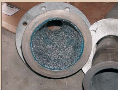
Paper Recycling Mill Cyclone
