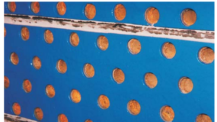
CeramAlloy CL+ applied to complete the project.
