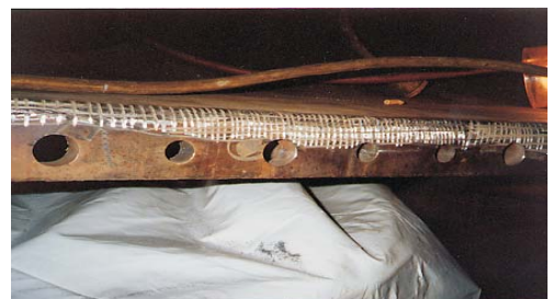
Smooth, ¼ inch thick aluminum angle coated with ENECON
