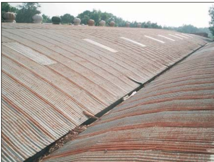
Note the holes in roof.
