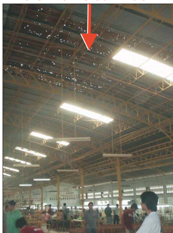
Note the holes in roof.
