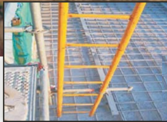
SuperBond Sprayed Over Existing Concrete & Reinforcing Bar.
