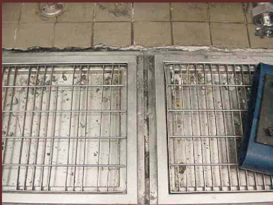
Portions of tiles where grout had failed were chipped away.
