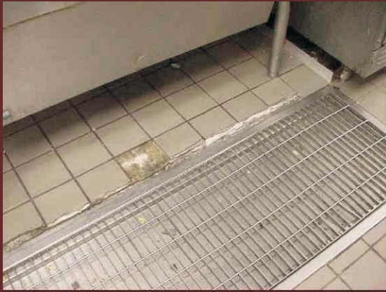
Portions of tiles where grout had failed were chipped away.
