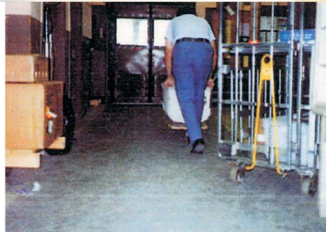
DuraQuartz providing years of trouble-free performance at Postal Center loading area.
