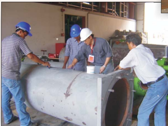
DurAlloy being applied to repair pitted areas.
