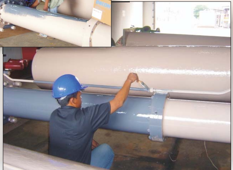
Final coat of CHEMCLAD SC being applied.
