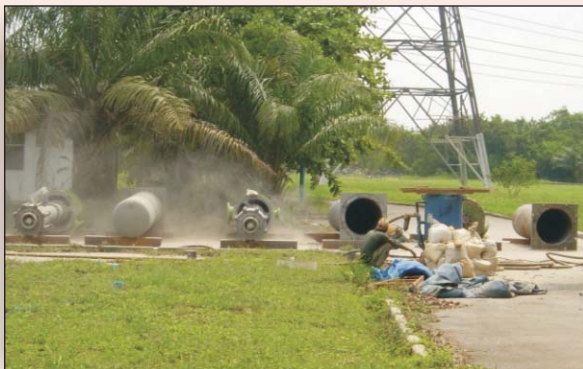
All pump sections were grit blasted.
