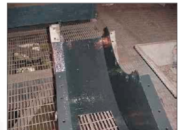
Two coats of CHEMCLAD XC were applied to all interior surfaces and flanges.
