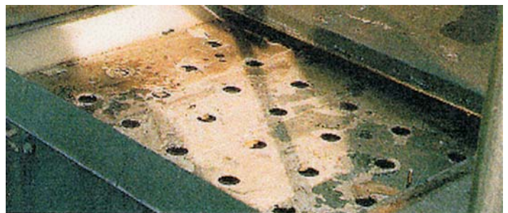
Pool paint peeling on pans poses problems.
